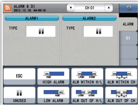
Fig. 45) Alarm selection screen
